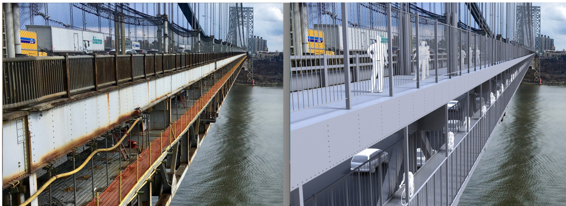
Another configuration would replace the temporary catwalk beneath the walkway with a permanent bikeway. Image: Neile Weissman, Joseph Lertola
