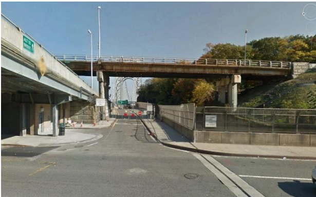
Existing condition at NJ-South: Hudson Terrace looking east: absence of crosswalk, entry area and street buffer; narrow sidewalk with vehicular gate impediment
