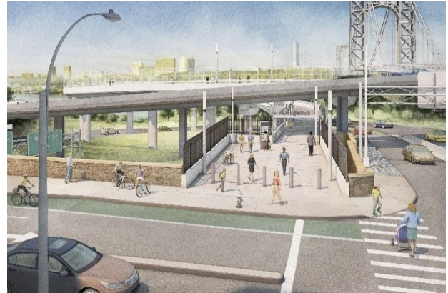
Future view at NY-South: south sidewalk pedestrian operation includes a spacious entry plaza, viewing platform and main span access ramp
