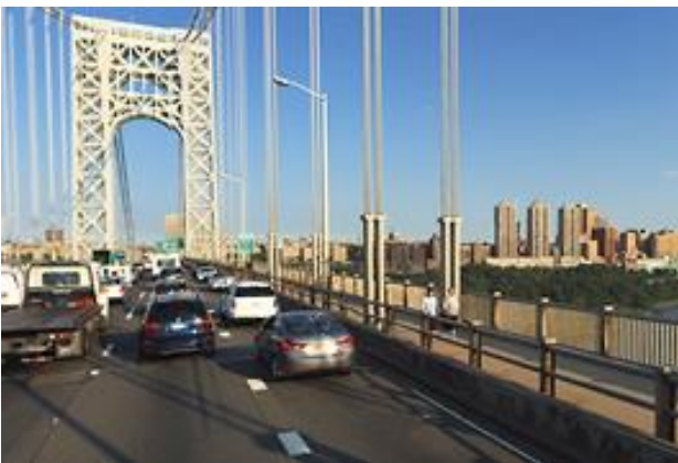
Partial height fence at the approach ramps and main span
