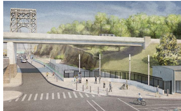
Future view at NJ-South: south sidewalk pedestrian operation includes a new crosswalk (along Hudson Terrace), spacious entry plaza and main span access sidewalk
